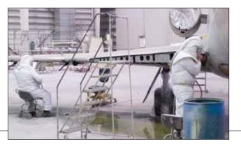
control surfaces and thickness requirements for various fuselage areas. Attention and care devoted to surface preparation increases the coating's protection level and lengthens its useful life. Masking is also important to protect composite components from stripping chemicals and to avoid crazing on windows and windscreens, contamination of actuators and other moving parts
